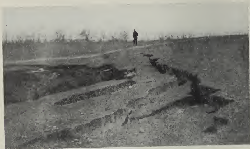
FIG. 10.—Cracks and breaks due to shear. View along the rim of a large pit hole caused by an extensive movement into a shallow mine. In the right foreground the mass of earth has dropped 18 inches.
